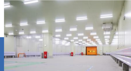
Temp. Controlled Room (+1°C~+20°C): 993㎡
